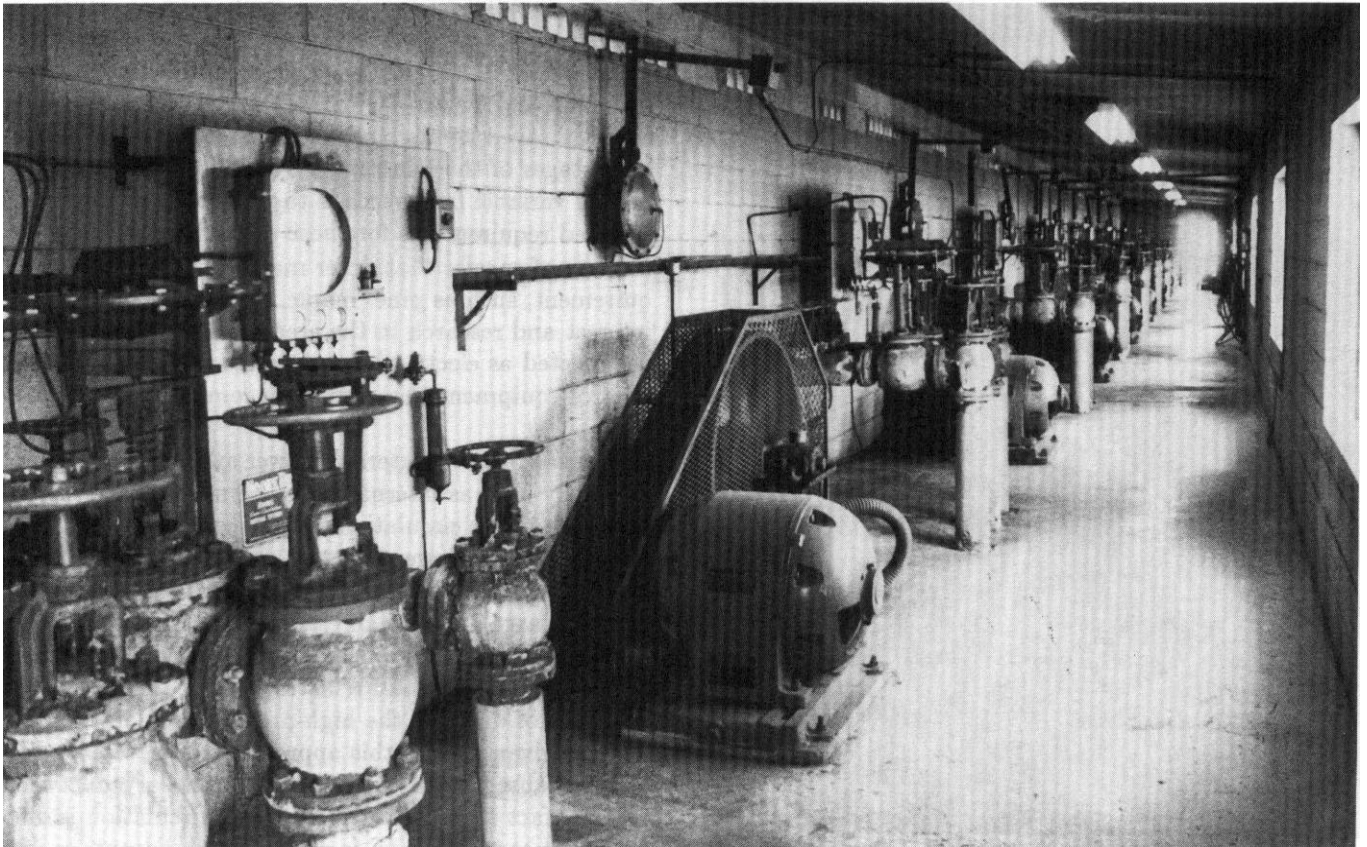
Figure 2-17—Control room for battery of lineshaft kilns, showing motor and pulley on lineshaft, recorder-controller, air-operated control valves to headers,
